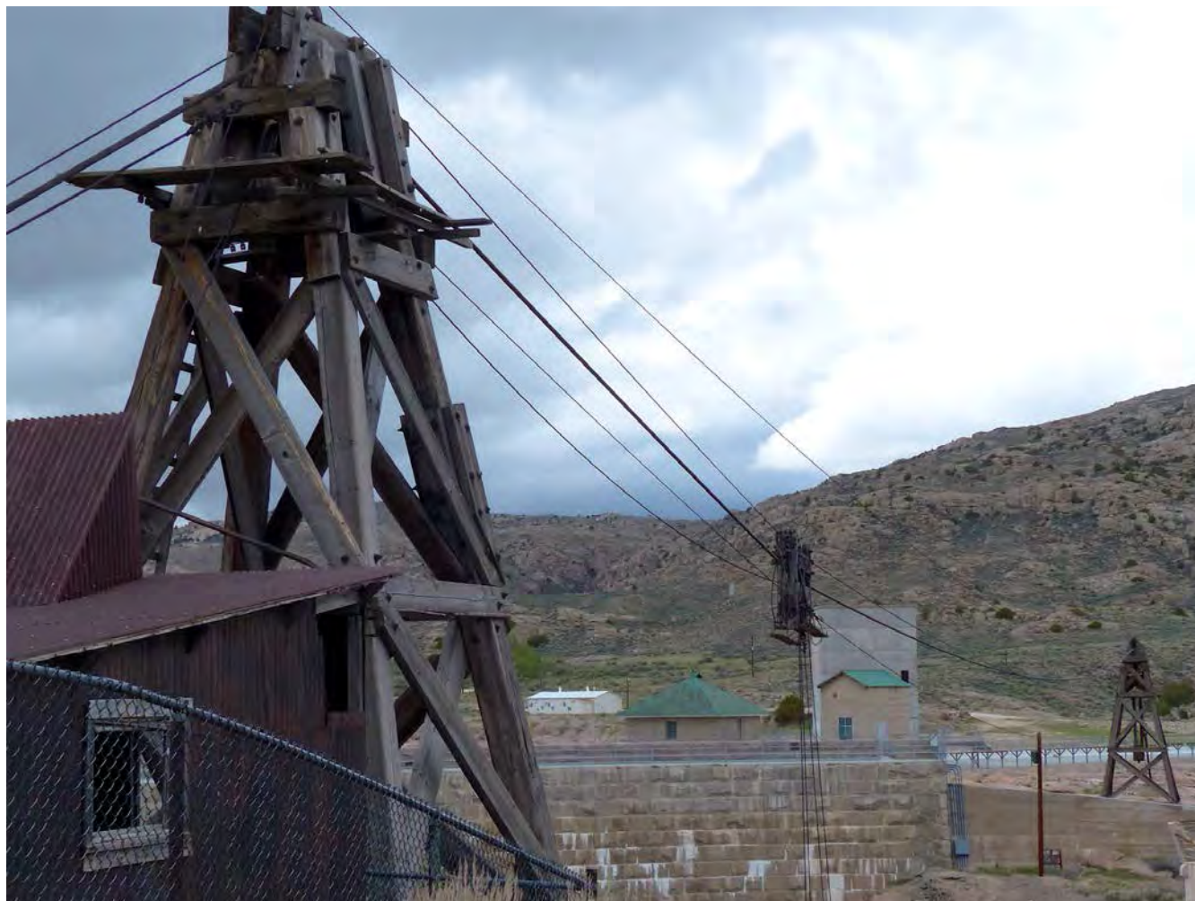
Photo #20: Long view of 1920 cableway system. From the left, cableway powerhouse, south tower, carriage cable and bucket hook system, and north tower. (Features M and N, contributing). Camera facing northwest.
