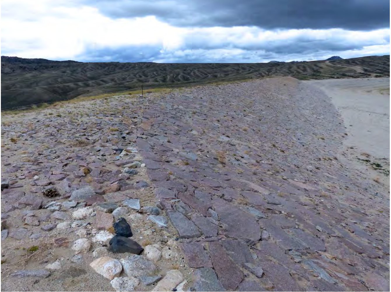
Photo #21: Pathfinder Dike (Element 2, contributing). Note hand placed granite rock protective facing on the upstream (right) side of the dike. The rubble rock visible on the downstream face is part of the earthen/rock matrix of the dike embankment. See historic photo #20 showing placement of the protective rock in 1910. Camera facing south from north end of the dike.
