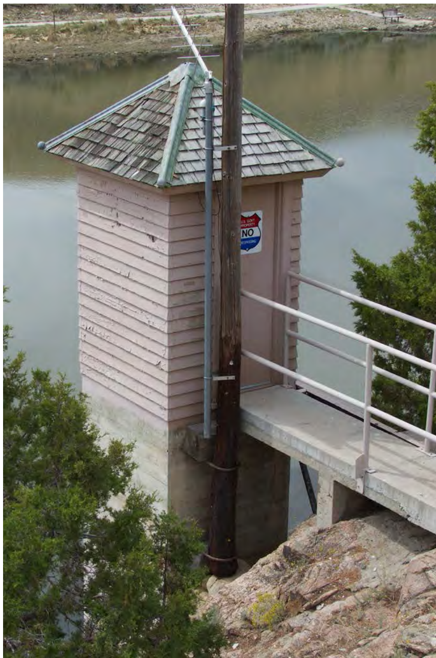
Photo #49: North and east elevations, Stream Gage Station instrument house and concrete stilling well (Element 6, contributing). Camera facing southwest.
