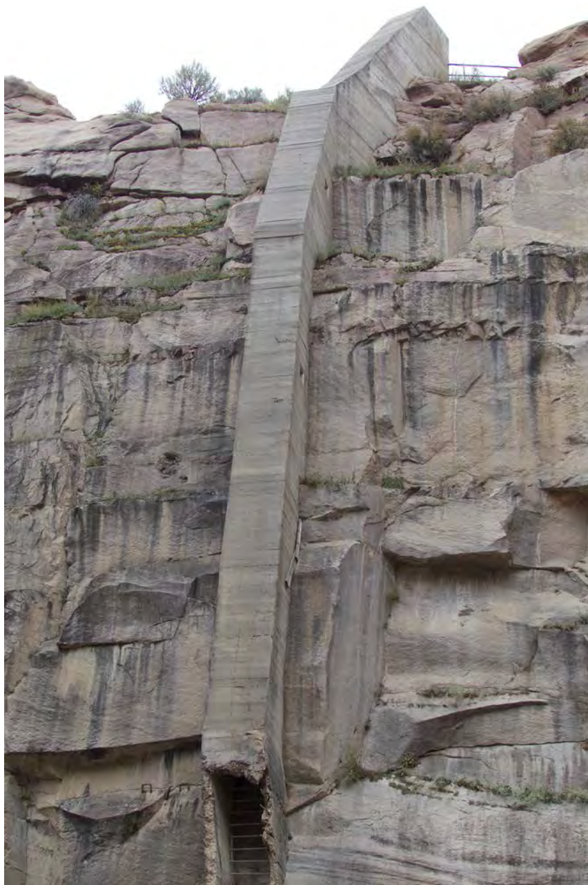
Photo #45: Abandoned concrete access ladderway (Feature G, contributing) from canyon floor. Note rebar used as ladder rungs. Camera facing south.
