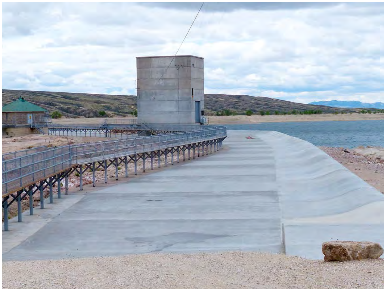
Photo #7: New spillway ogee weir and concrete apron, completed in 2012, Fremont Canyon Fixed Wheel Gatehouse, and Emergency Gatehouse. Camera facing south.
