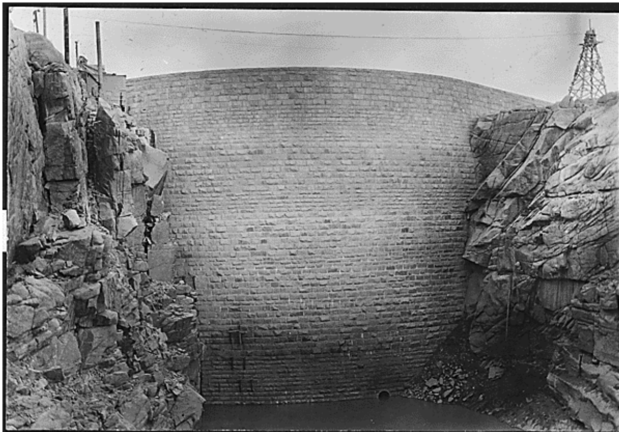
Historic Photo #18: October 19, 1909, Pathfinder Dam, upstream face. Old cableway system north tower in upper right corner
