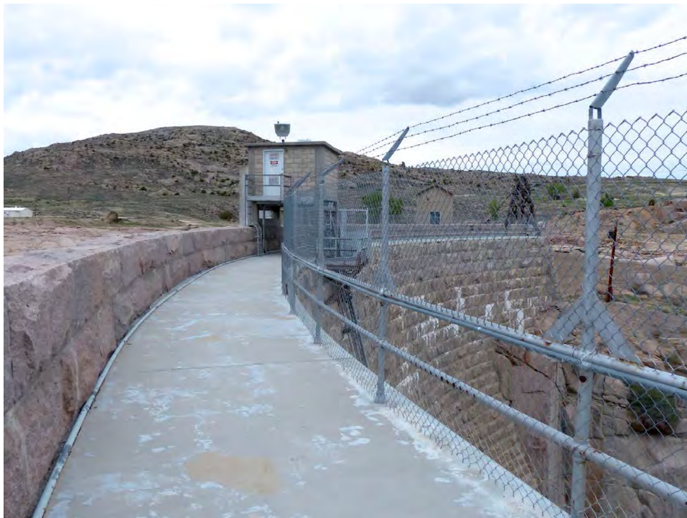
Photo #14: Pathfinder Dam crest, note safety fencing on right and parapet wall on left, and elevator machine house. Sluice Gatehouse and north cableway tower are immediately to the right of elevator machine house. Camera facing north.
