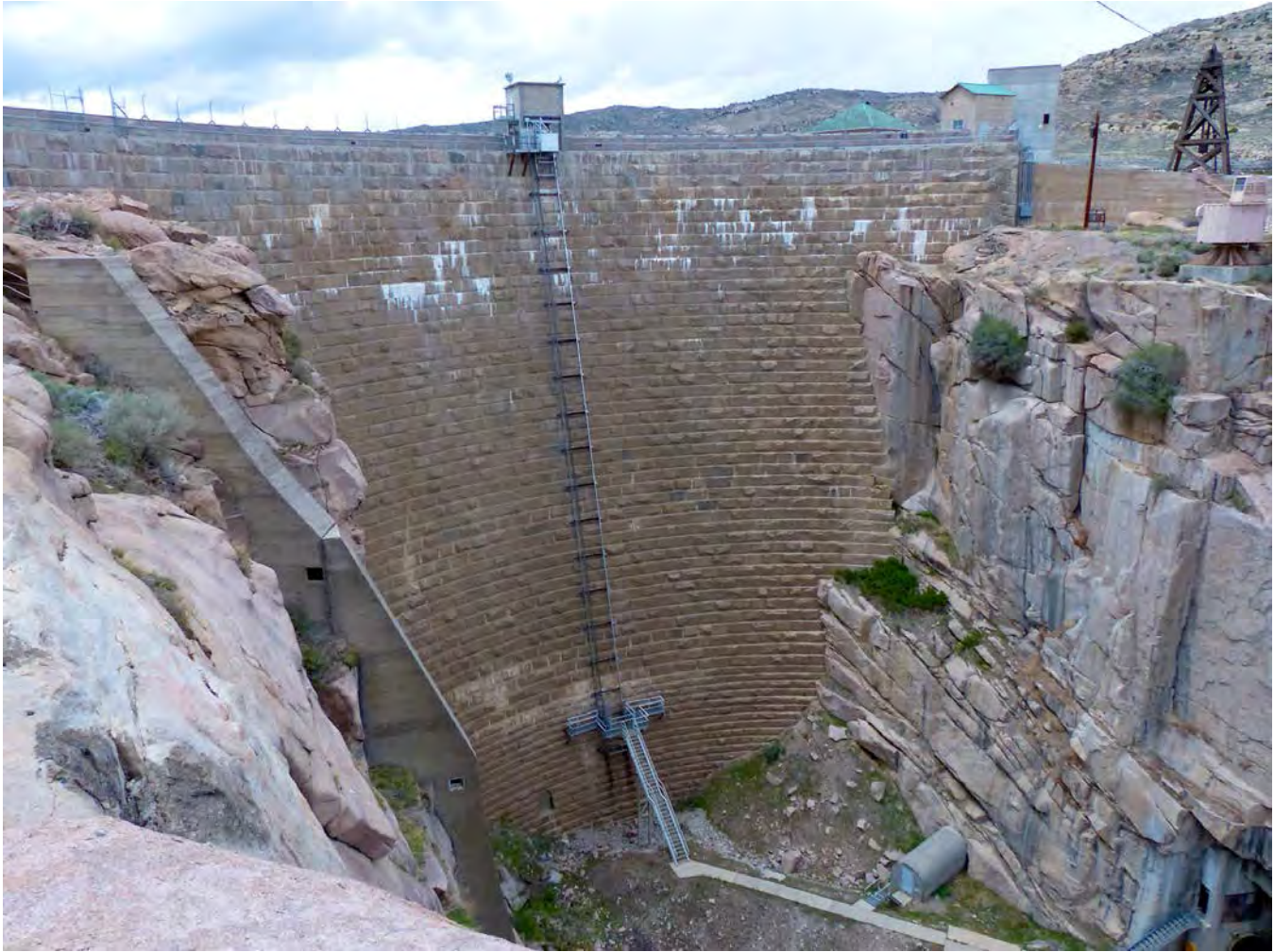
Photo #3: Pathfinder Dam, camera facing northwest. Note south access ladderway on canyon wall in the left of the photo (Feature G, contributing). Also note the elevator and associated ladder and walkways (collectively Feature B, non-contributing) leading to high-pressure gate access structure (Quonset hut) and river outlet control house in the lower right corner of the photo (both part of Feature E, non-contributing).
