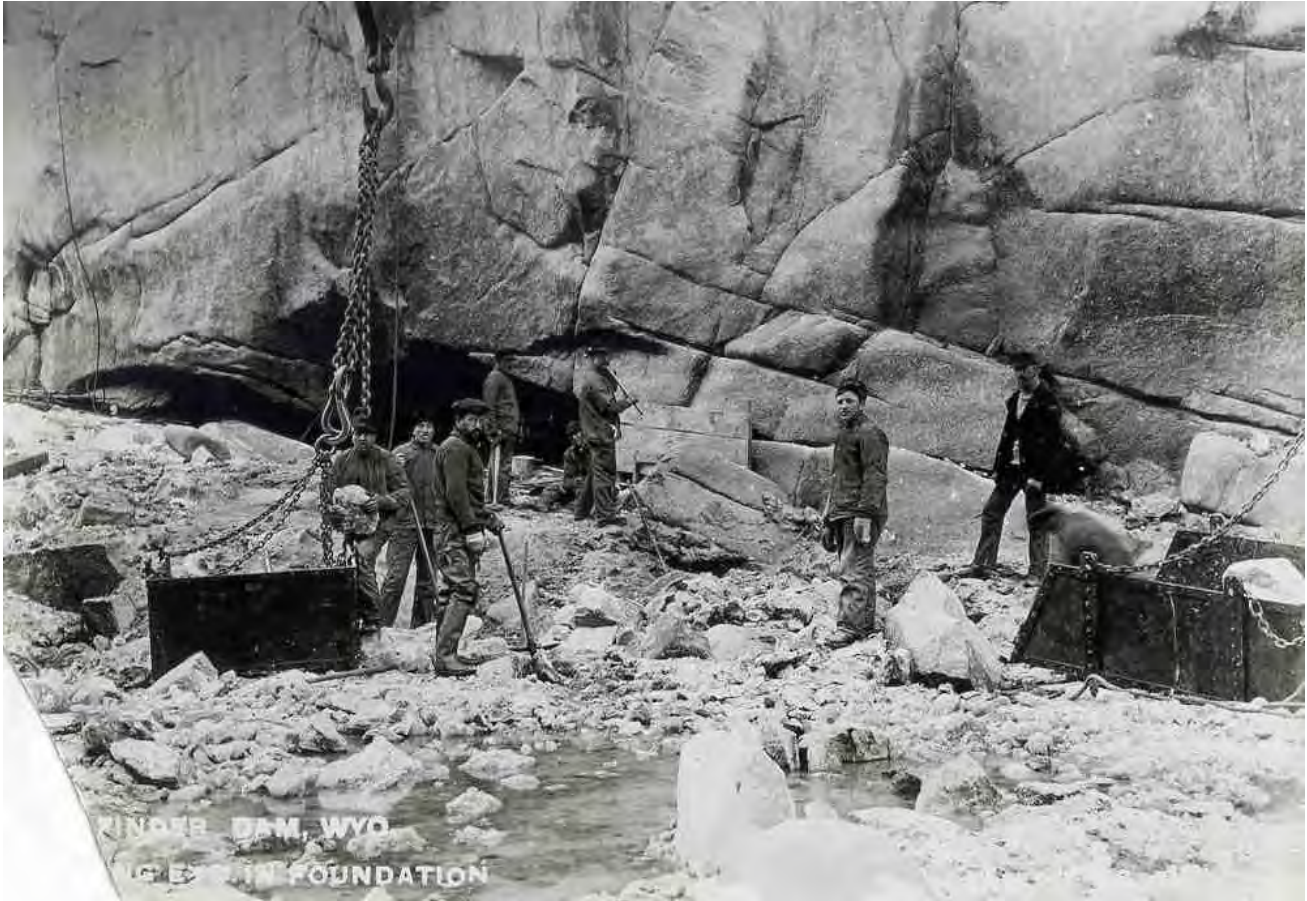
Historic Photo #3: View taken January 23, 1906, and shows starting of excavation for the dam's foundation. All loose material was removed and the top of the rock removed to a sound bedrock foundation only 10 feet below the ground surface.
