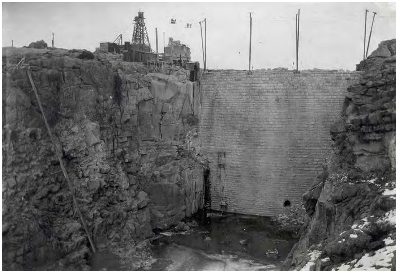
Historic Photo #13: 1908, Pathfinder Dam upstream face. North towers of original two cableway systems shown. Note exposed access ladder on left hand side of canyon, precursor to the enclosed ladderway built a few years later. Emergency Gatehouse under construction (structure immediately next to dam).
