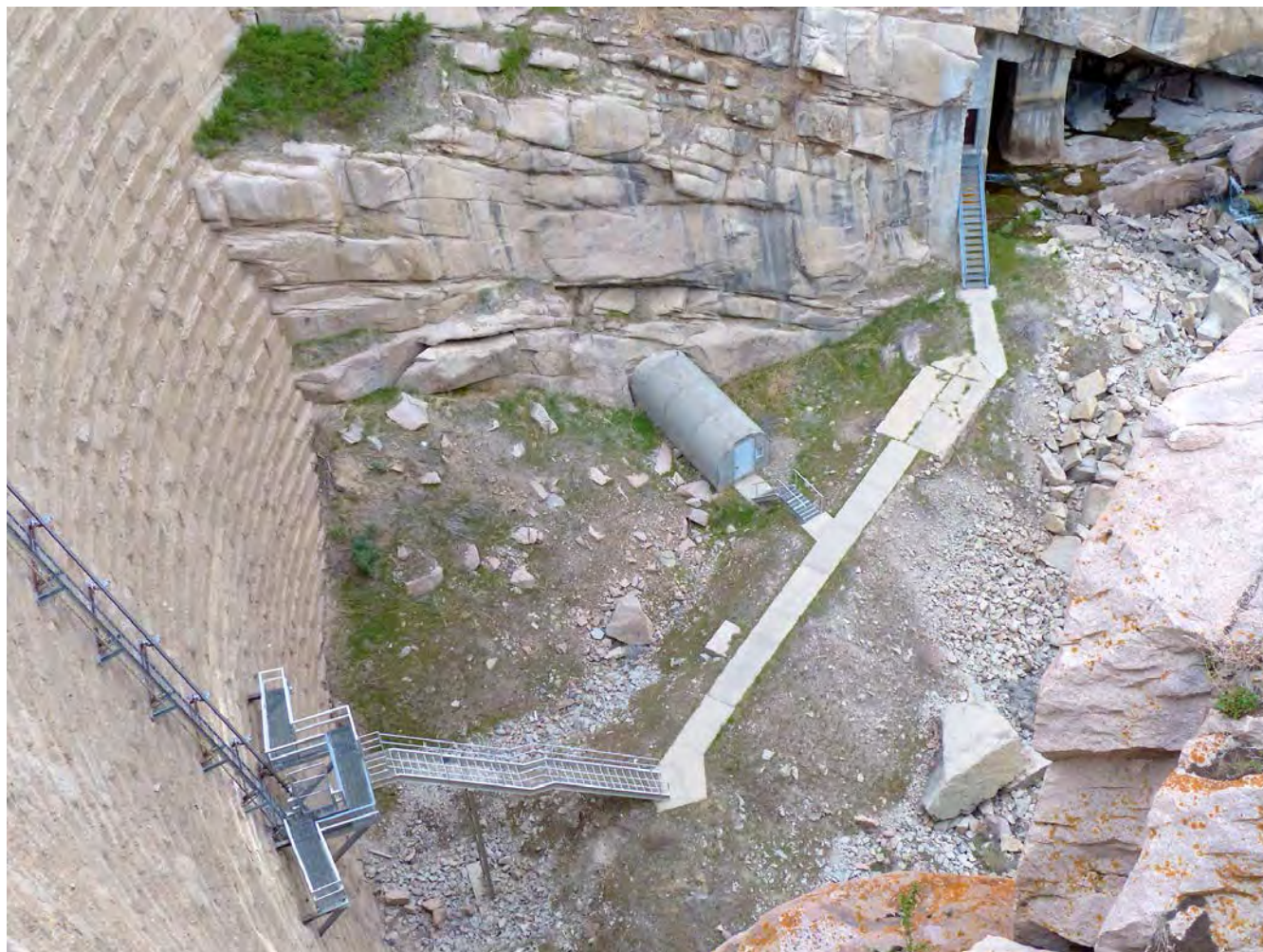
Photo #11: View from above of (from left) the dam's downstream face, the elevator track, walkway, and the high-pressure gate control (Quonset hut) access structure. Camera facing down and northeast.
