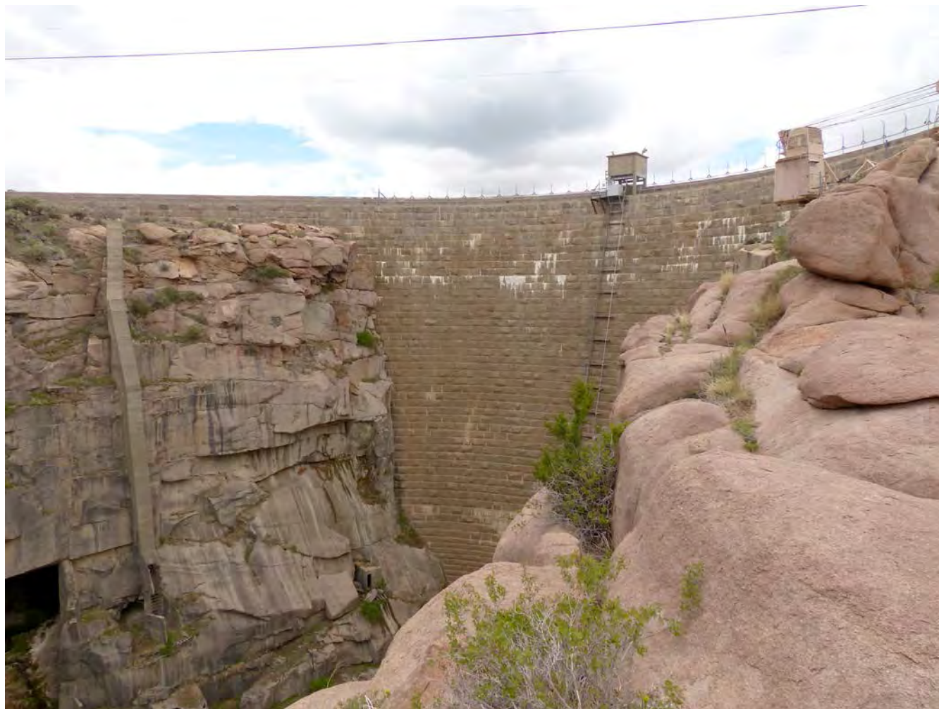
Photo #4: Pathfinder Dam, south access ladderway (Feature G, contributing), and south tunnel outlet and auxiliary tunnel balanced valve control house (both elements of Feature F, non-contributing). The south tunnel outlet is the large opening visible to lower left of the ladderway; the value house is the small structure in the rock face to the right of the ladderway. Camera facing southwest.
